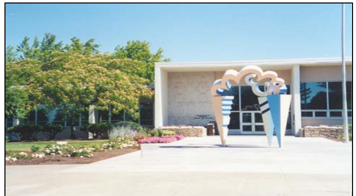
Sonoma County Administration Building
